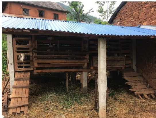
Goat Shed Construction
