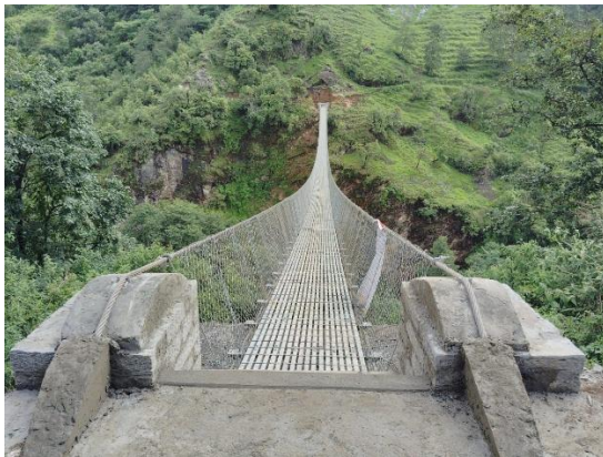
Trail Bridge Construction
