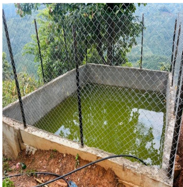
RCC tank built on POG irrigation activities
