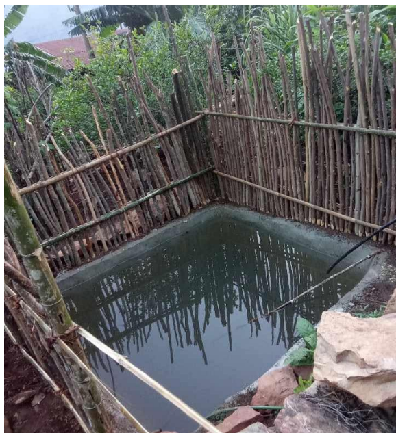
Construction of Soil Tank
